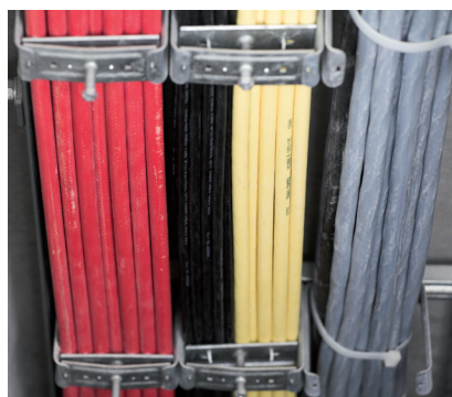
Triax, video and audio cables made by Draka Communications – extreme space ratio and still optimal transmission characteristics.
